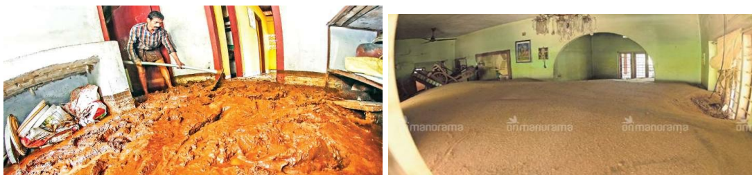
Figure 13:44 Photos of sediment deposited in houses as the result of flood
