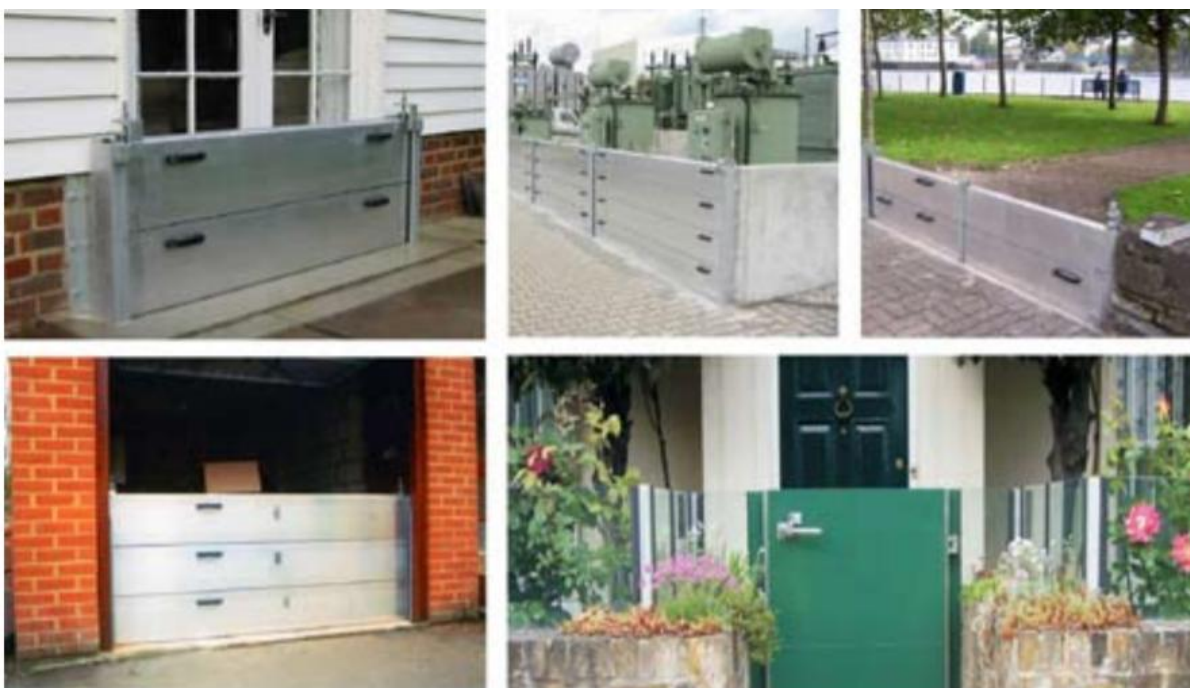
Figure 19:12 Dry Flood Proofing Techniques
