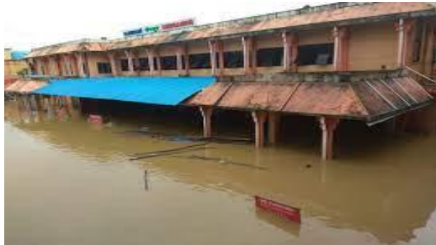
Figure 13:47 Chengannur Railway Station during Flood 2018
