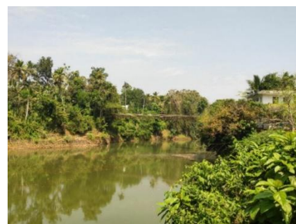
Figure 21:20 Existing Hanging bridge
