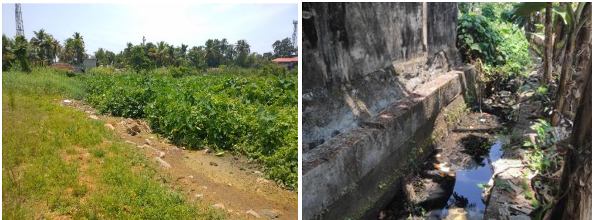
Figure 23:2: Existing condition of Vettuthodu
