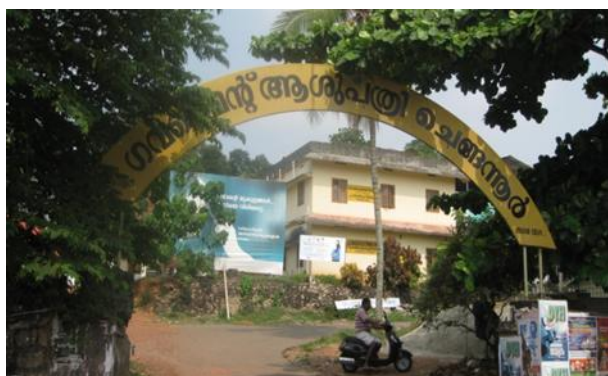
Figure 10:4 Govt Hospital Chengannur
