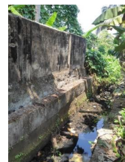
Figure 21:25 Existing Condition of Vettuthodu
